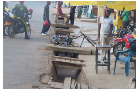
Streets with open drains
