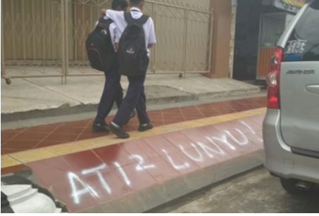
Use of slippery ceramic tiles on footpaths
